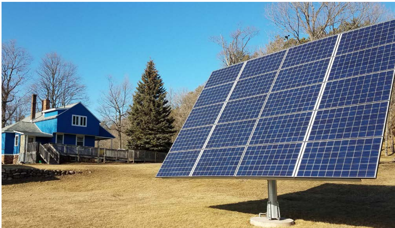
Ground-mounted monopole SES. Photo by Bradley Neumann.
